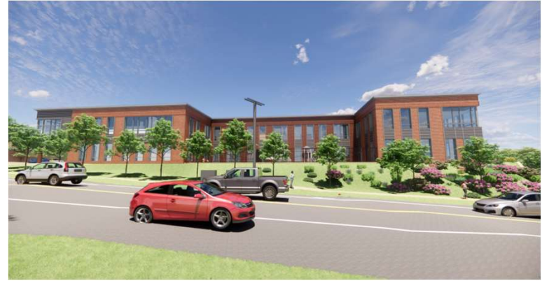
View Along Layton Hall Drive
