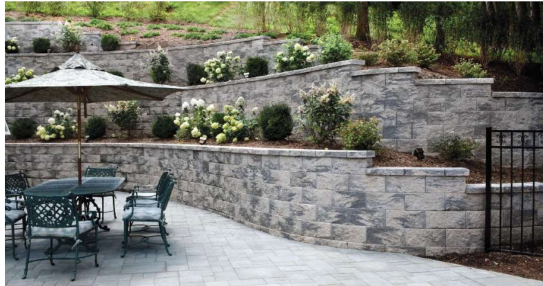
Stone wall terracing
