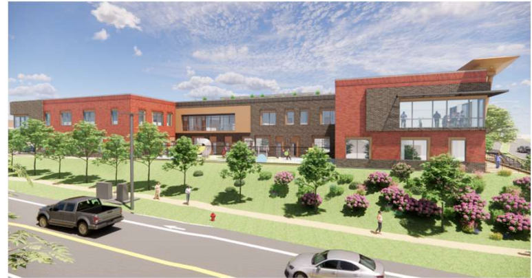
View Along Layton Hall Drive
