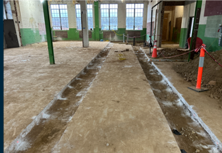
MEP Under-Slab Work
