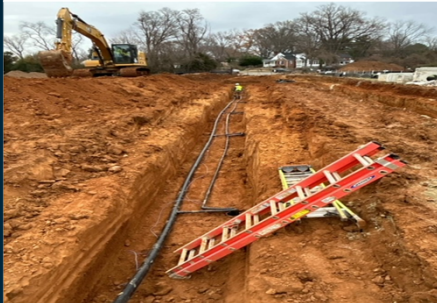
Geo-Thermal Well –Horiz. Loop Install
