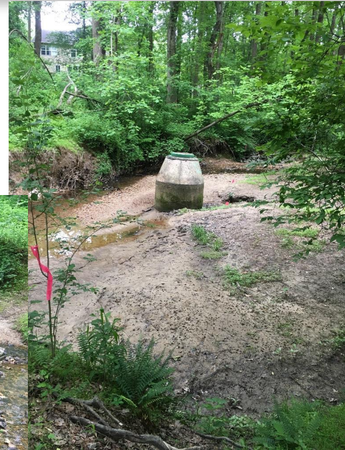
Exposed sanitary sewer
