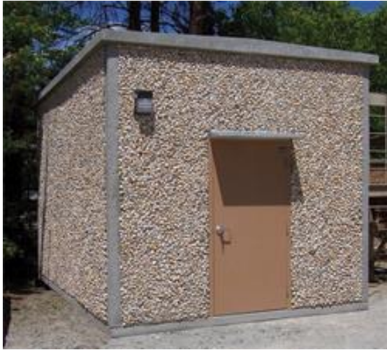
Typical Utility Shed (Existing)
