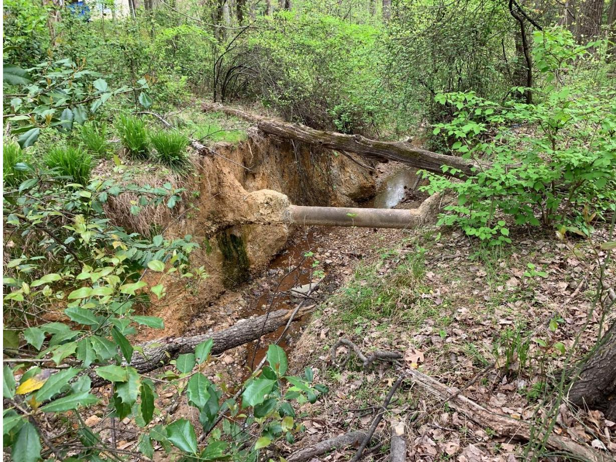
Exposed sanitary sewer pipe
