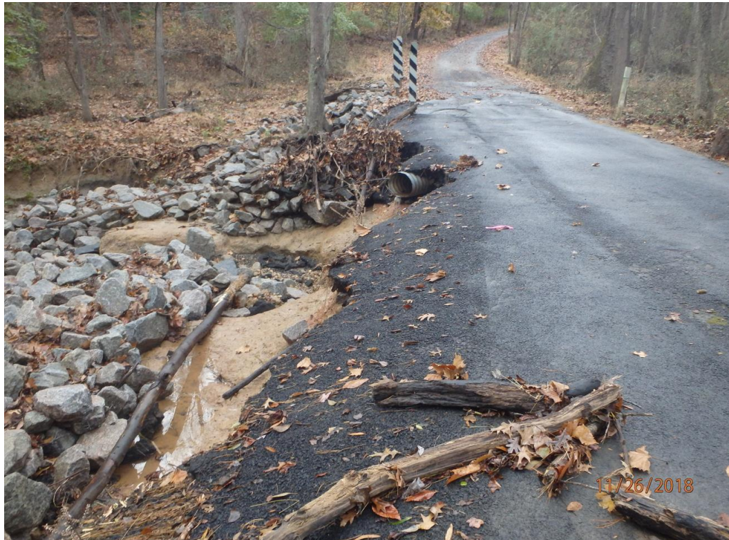
Figure 2. Existing Hickory Hollow Lane crossing of Rocky Branch.
