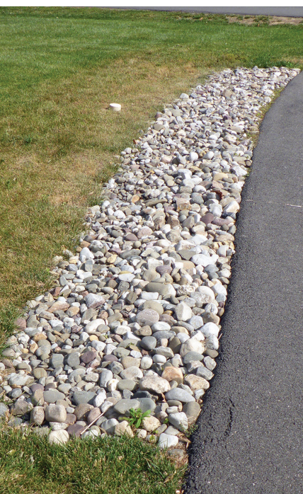
The OBSERVATION WELL is the white pipe with a cap located to the left of the trench surface. The INFLOWS are the lawn and the driveway.
