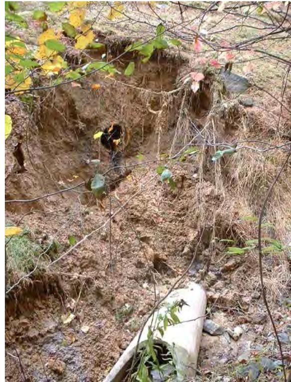
*Photo 3.55 Severe erosion and pipe segment separation at a 16-inch outfall located near Alexander Bell Drive (DFSB006.P006).*
