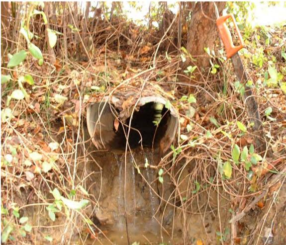
*Photo 3.1 Erosion at the end of stormwater pipe located off of Collin Farm Land (DFCH021.P003).*
