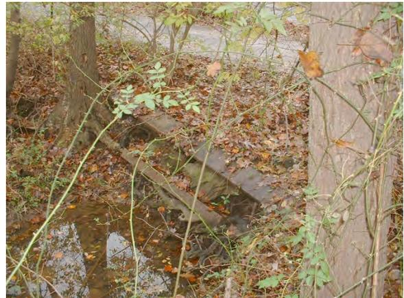
*Photo 3.109 Pipe culvert at the headwaters of Angelico Branch. This is the only crossing in the watershed that has more than a moderate impact on the stream. (DFAB002.C003)*
