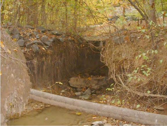
*Photo 3.56 An 18-inch outfall causing severe erosion located downstream of the outfall shown in Photo 4.1 (DFSB006.P005).*
