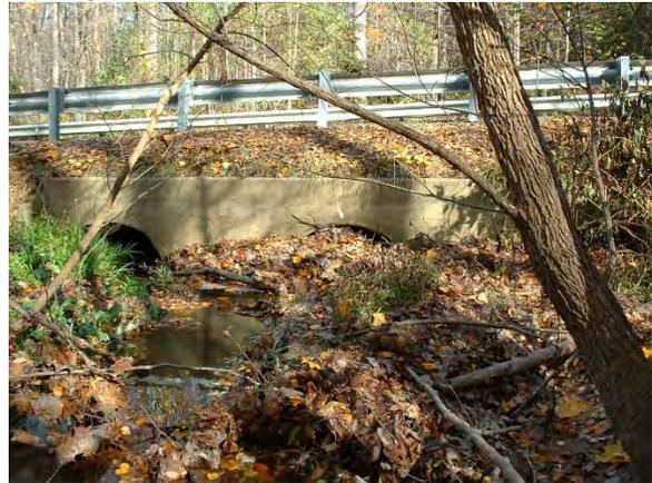
*Photo 3.94 Crossing under Fox Mill Road north of Shady Mill Lane. Crossing has excessive sedimentation (DFLD015.C002).*
