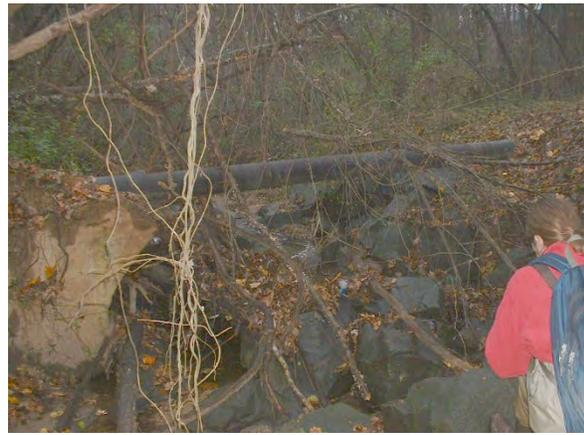
*Photo 3.89 Sanitary line crossing the stream above the baseflow (DFPB010.U001).*
