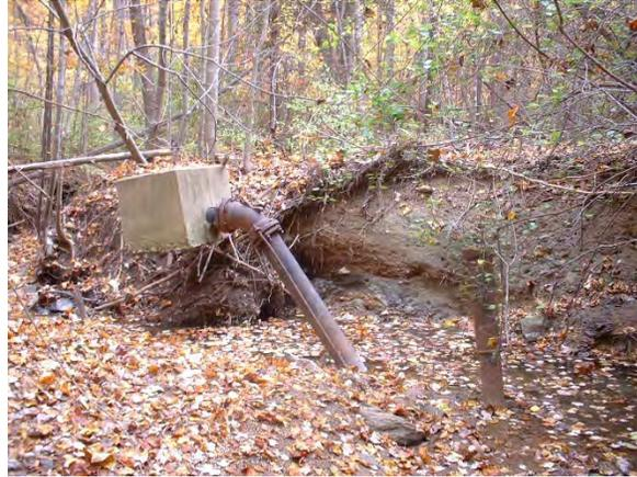
*Photo 3.57 Pipe located south of Sunrise Valley Drive and just east of Barton Hill Road. Major erosion around the structure is evident (DFSB006.P003).*
