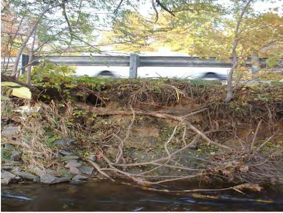
*Photo 3.26 Severe erosion that could pose a threat to road safety along Route 7 to the east of Carpers Farm Way (DFCR001.E001).*
