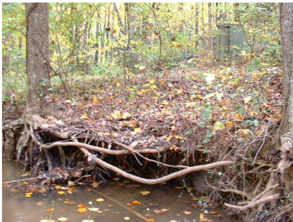
Photo 3.67 Erosion north of Lawyers Road near Pinoak Lane (DFGL006.E001)
