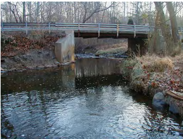
Photo 3.52 Colvin Run Mainstem at Hunter Mill Road
