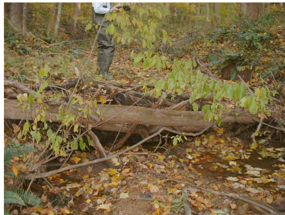
Photo 3.40 Obstruction located between Tebbs Lane and Cilicia Street (DFRR001.T002).
