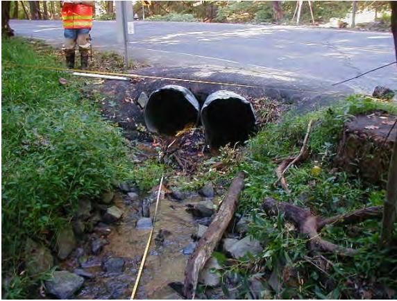
Photo 3.113 Angelico Branch at Lawyers Road
