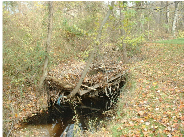
Photo 3.79 A severe obstruction located upstream of Chain Bridge Road near Echols Street (DFWC028.T001).
