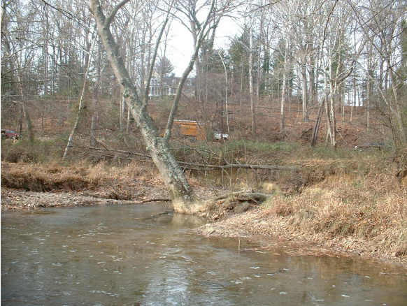
Photo 3.140 Roadway buffer encroachment near Waples Mill Road (DFDF034.B001).
