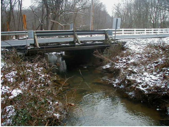
Photo 3.20 Piney Run Mainstem at Walker Road
