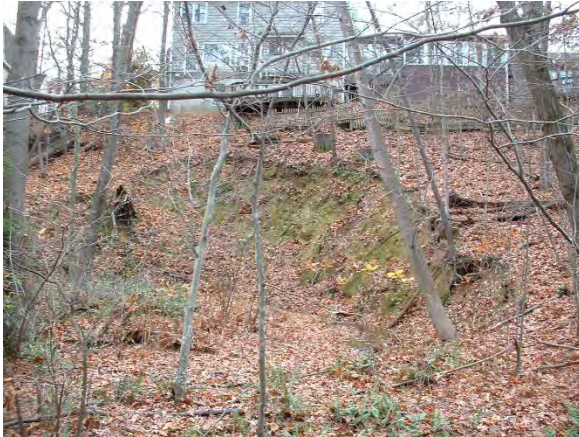
Photo 3.118 Eroding bank located in the southern edge of the Difficult Run Stream Valley Park in the Clarke's Landing subdivision directly north of the terminus of Timberline Court (DFSF002.E001).
