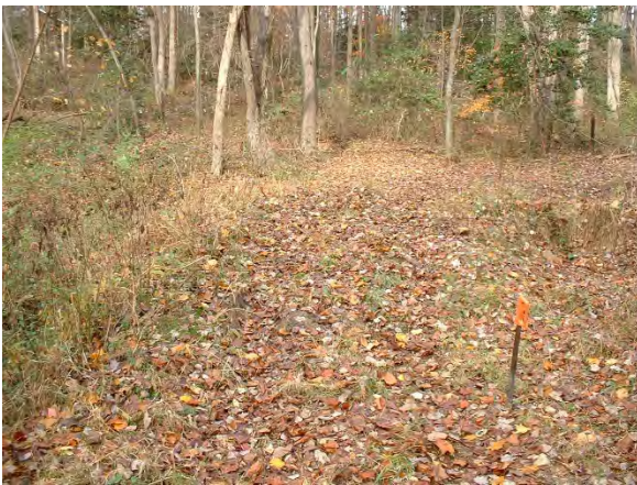
Photo 3.5 Earthen berm located in the upper reaches of Captain Hickory Run near Thunderhill Court (DFCH009.T001)
