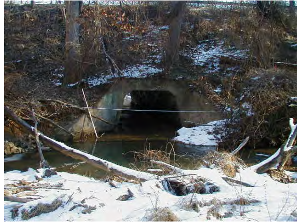
Photo 3.44 Culvert 79 on Rocky Run mainstem at Old Dominion Drive
