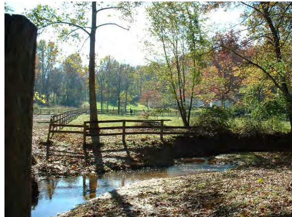
Photo 3.101 Buffer impact in the Hollybrook community, directly north of the terminus of Hollybrook Place, mainstem of Little Difficult Run (DFLD003.B002).
