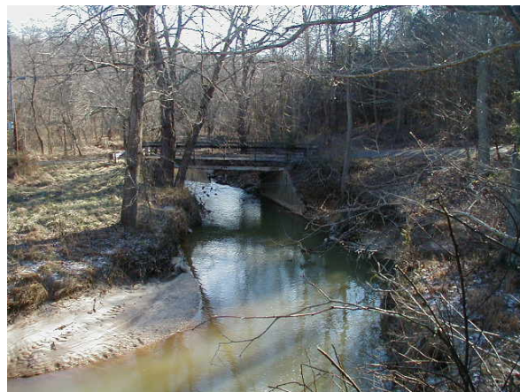
Photo 3.149 Difficult Run Mainstem at Vale Road
