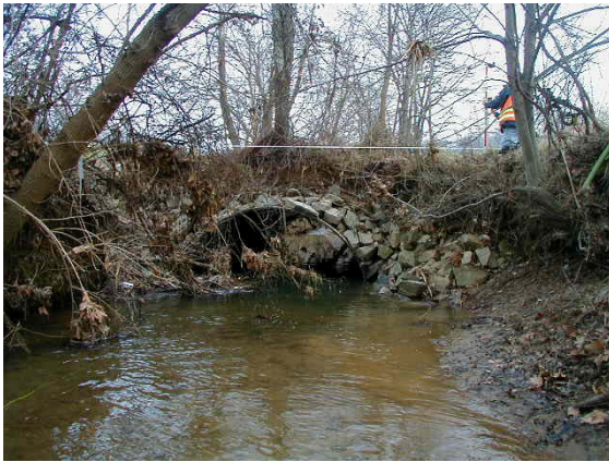
Photo 3.31 Lower Difficult Run Mainstem along Leesburg Pike
