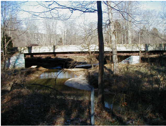
Photo 3.150 Difficult Run Mainstem at Vale Road
