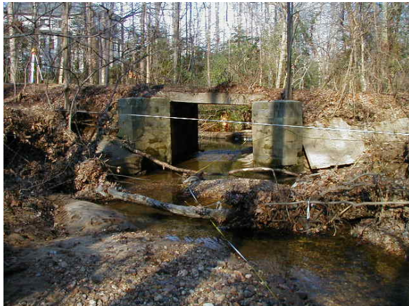
Photo 3.86 Crossing at Northern Neck Drive (DFOR701.T001).
