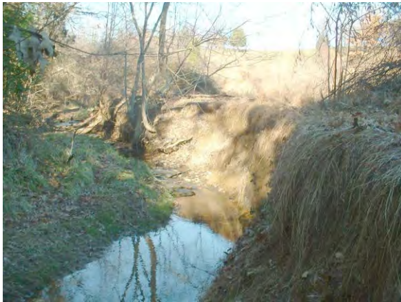
Photo 3.70 Eroding channel located between Brittenford Drive and Hunt Country Lane (DFDF049.E002).
