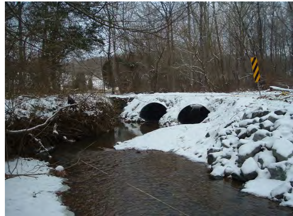
Photo 3.42 Culvert 75 at Bellview Road on Rocky Run mainstem.
