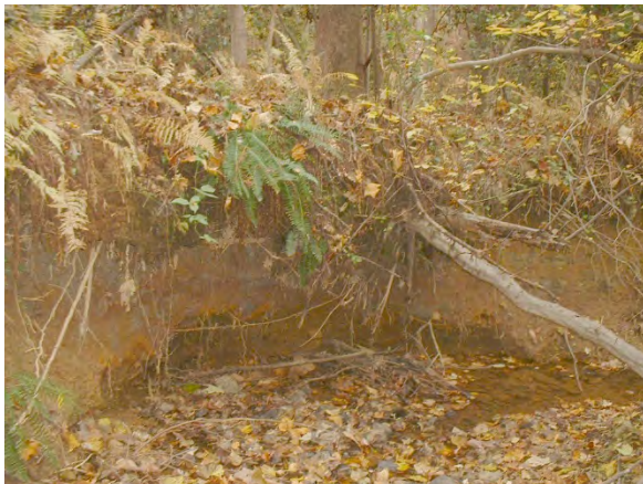
Photo 3.50 Obstruction just upstream of Lake Fairfax to the west of Aldenham Lane (DFCR013.T001).
