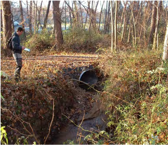
Photo 3.24 Located near Leigh Mill Road has downstream and upstream bank erosion and minor bed erosion (DFDF019.C001).
