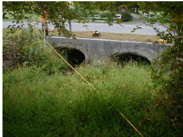
Photo 3.143 Difficult Run Tributary at Valley Road
