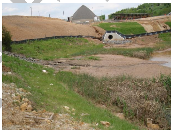
Figure 2-41: Erosion and heavy sedimentation in several ponds southeast of the intersection of I-66 and Fairfax County Parkway
