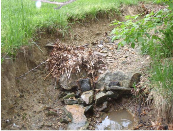
Figure 2-20: Severe erosion occurring at the end of a concrete trickle ditch in the Little Rocky Run subdivision (Battle Rock Drive)
