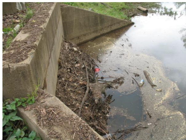
Figure 2-40: Obstruction in pond near Tractor Lane
