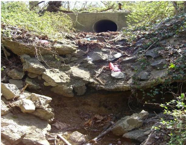
**Figure 4-9: An eroded outfall**
