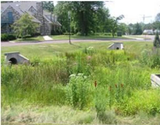
Figure 4-1: Dry stormwater pond
