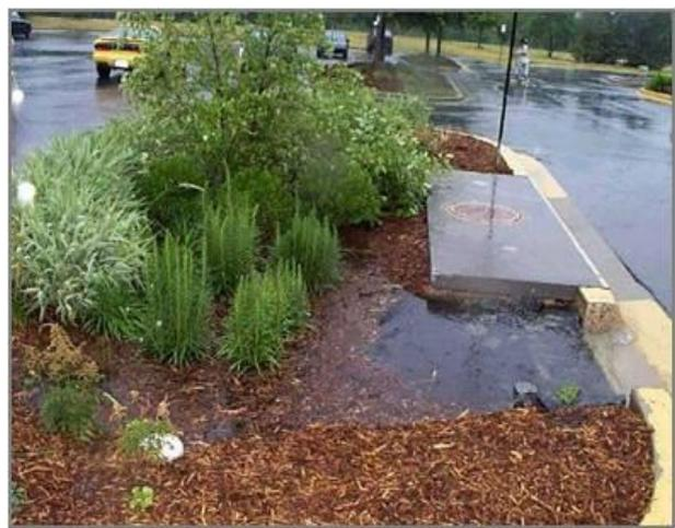
Figure 4-4: Parking lot bioretention filter
