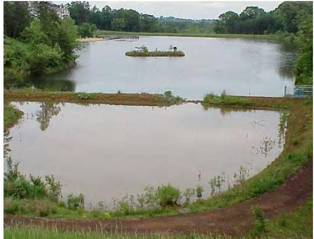
Figure 4-2: Wet stormwater pond with forebay
