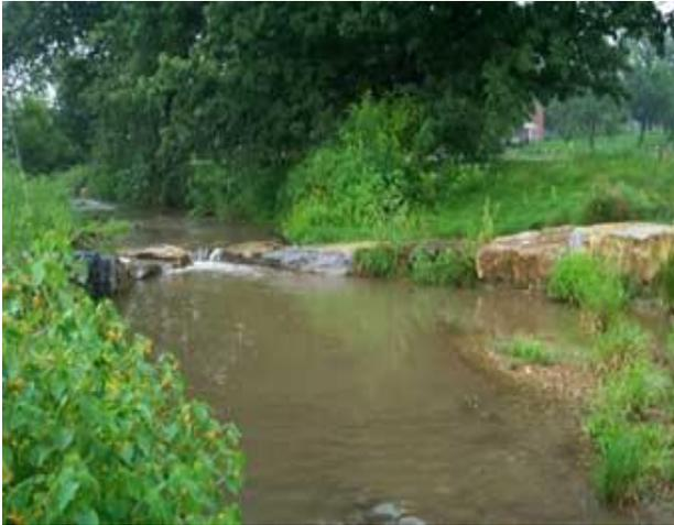
**Figure 4-7: Cross vane added to stream**
