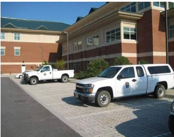
Figure 4-3: Parking lot pervious pavement
