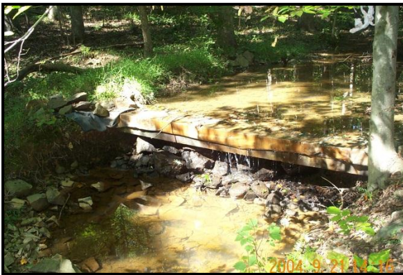
Homemade dam looking upstream
