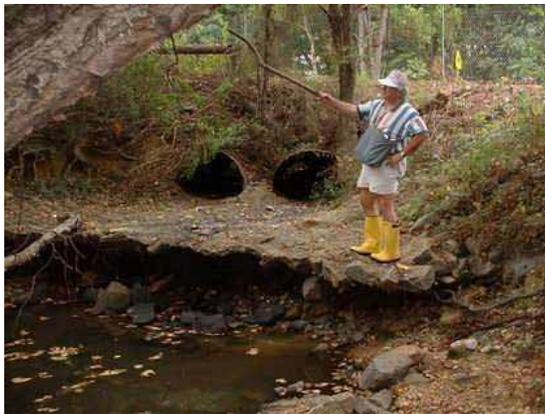
Photo 3.16 Severe erosion downstream of the Mary Baldwin Drive crossing
