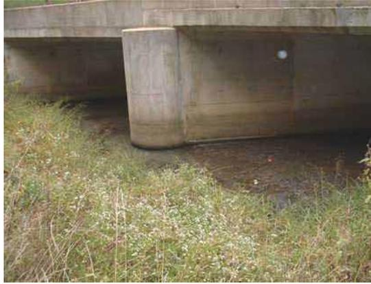
Photo 3.33 Four 10' x 15' concrete box culverts located under Collingwood Road to convey flows of the eastern tributary
