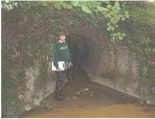
Photo 3.34 A 60" diameter concrete pipe outfall at the headwaters of the tributary to North Branch
