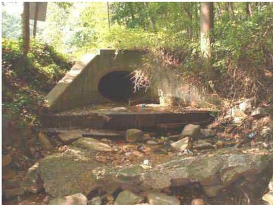
Photo 3.18 Discharge from 53"x 34" elliptical pipe outfall north of Devonshire Road caused moderate erosion on the downstream side
