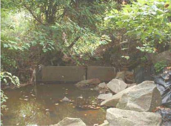
Photo 3.23 Concrete blocks obstructing the flow south of the intersection of Rollins Drive and Radcliff Drive
