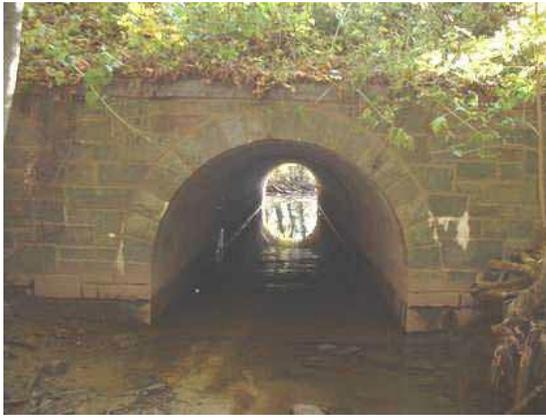
Photo 3.41 Concrete arch culvert of size 7' by 6' located under George Washington Memorial Parkway
