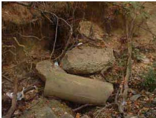
Photo 3.19 Severe erosion caused by discharge from an 18" pipe outfall west of the Mary Baldwin Drive crossing
