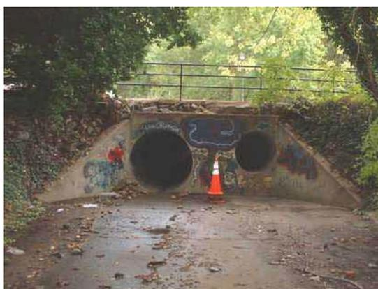
Photo 3.11 5' and 3' diameter pipes located under Linton Lane
