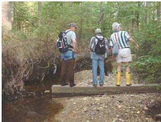
Photo 3.21 Minor erosion of the right bank at the ditch outfall north of the intersection of Paul Spring Road and Pickwick Lane
