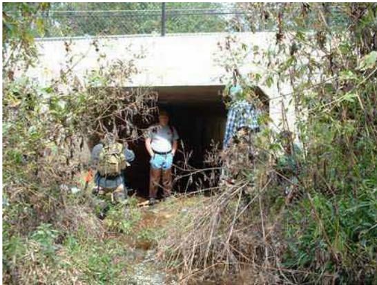
Photo 3.32 Five 12' x 8' concrete box culverts located under Collingwood Road to convey North Branch main stem flows
