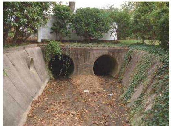
Photo 3.13 Double 3' (diameter) concrete pipes located west of Vernon View Drive
