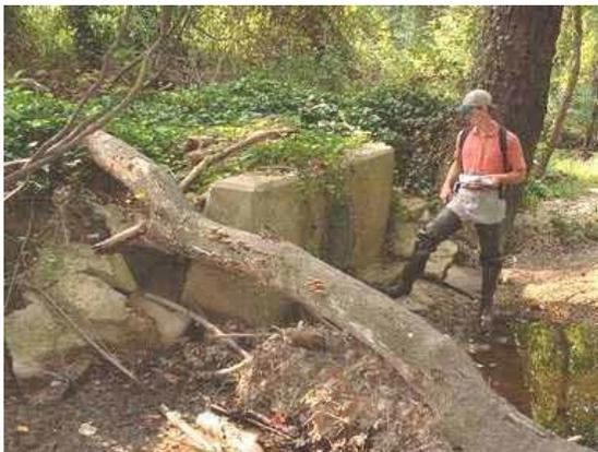
Photo 3.20 Severe erosion caused by discharge from 24" pipe outfall located north of Wellington Road
