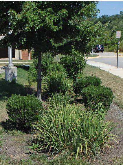
**BIORETENTION FACILITY** showing the ponding area, mulch layer, trees, shrubs, and overflow containment berm; the **INFLOW** is the grass area located to the right of the ponding area.
