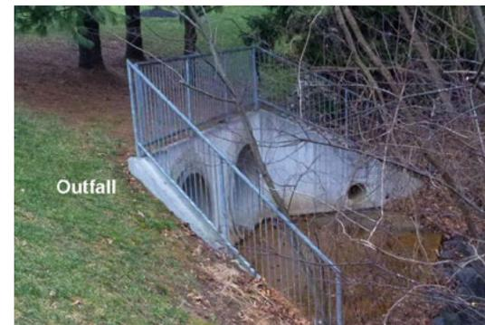
**EXTENDED DETENTION (DRY) PONDS** do not hold a permanent pool of water across the pond floor. Runoff is temporarily stored in the extended detention pond floor. They may be enhanced to include micropools at the inflow structure, sediment forebays with permanent pools and deep pools or wetland cells to improve water quality. Extended detention dry ponds provide both water quality and stream protection benefits.
