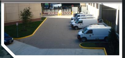
The PSHQ service driveway is paved with permeable pavers. These interlocking brick pavers allow water to drain through the gaps between the bricks into a gravel base below. The water then infiltrates or slow flows into the storm drain system that discharges to the wet pond.
