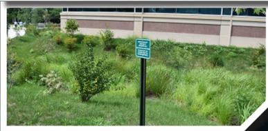
These depressed, landscaped gardens capture and filter stormwater runoff. During storms, runoff temporarily ponds then rapidly filters through a bed of sand, soil, and organic filtering media. Native plants like rushes and sedges help take up and treat stormwater, provide wildlife benefits, and create appealing landscaping.
