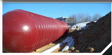
Rainwater is harvested from the top roof and collected in an underground, 25,000-gallon cistern. Water from the cistern is used to irrigate landscaping around the building.
