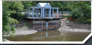
Using a cloud-based platform, the CMAC system continuously watches the weather forecast and monitors the pond water levels. The system automatically adjusts valves to meet site pollutant removal and volume control goals.
