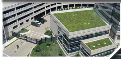
Five vegetated roofs use special drainage systems to slow down, evaporate, and filter rainwater before it enters the drain. Green roofs also moderate internal temperatures.
