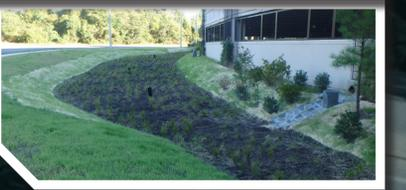
Vegetated swales provide the same services as bioretention cells, but they are shallower, configured as linear channels, and can be planted with sod or native plants. These swales create a 1,100-foot-long treatment path that terminates at an engineered outfall.
