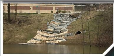
RSC systems (the outfall to the pond) is an open-channel, sand seepage filtering system that utilizes a series of shallow aquatic pools, riffle weir grade controls, native vegetation and underlying sand channel. The system combines features and treatment benefits of swales, infiltration, filtering and wetland practices.
