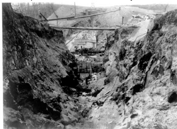
Construction of Lake Barcroft dam 1913-1915.
