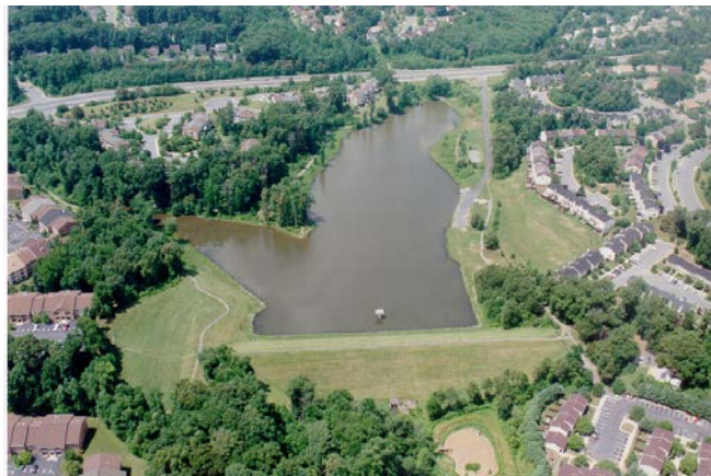
Lake Barton at Burke Centre, one of the six dams built as part of the Soil Conservation Service (PL566) pilot program.
