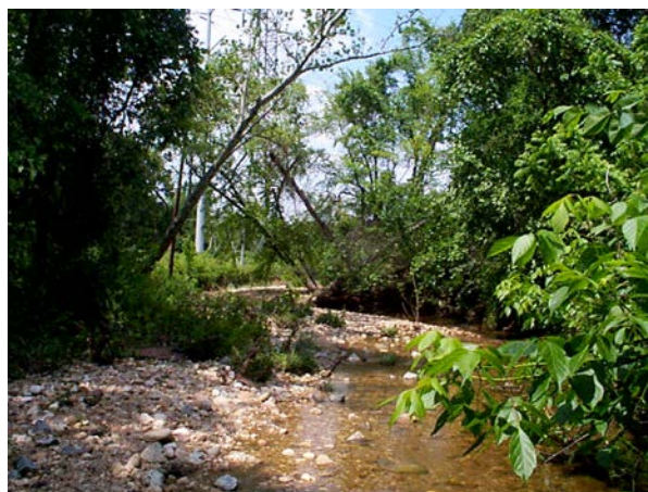
Tree falls are indicative of stream channel widening along Pikes Branch in the Cameron Run Watershed.
