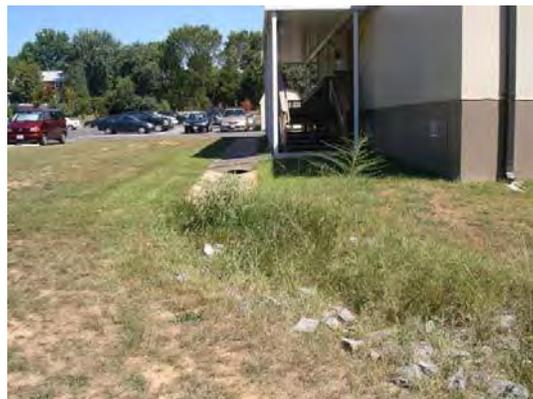
Convert concrete ditch to linear bioretention area and collect water from downspouts
