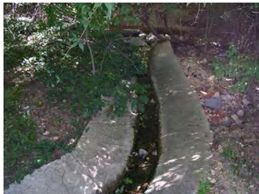
Divert flow from concrete channel into off-line bioretention area
