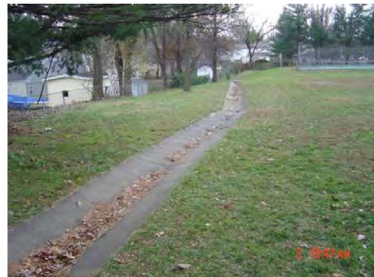
Convert concrete ditch to linear bioretention area
