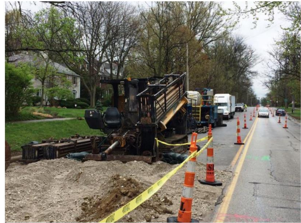
Figure 8. Example of HDD Within the Right-Of-Way
