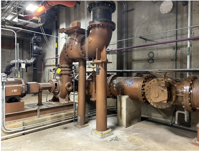
Figure 2-28: E2 Building Return Activated Sludge (RAS) Valve Replacement
