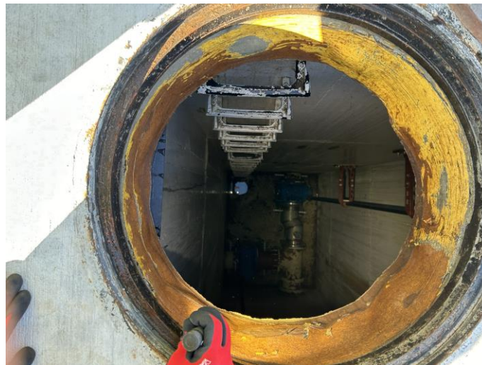
Figure 2-25: Circular Secondary Clarifier Isolation Valve Replacement
