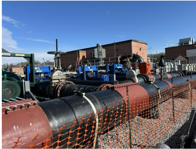
Figure 2-26: ASE Pump Station Bypass Pumping
