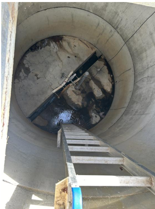
Figure 2-12: 3-inch Parshall Flume
