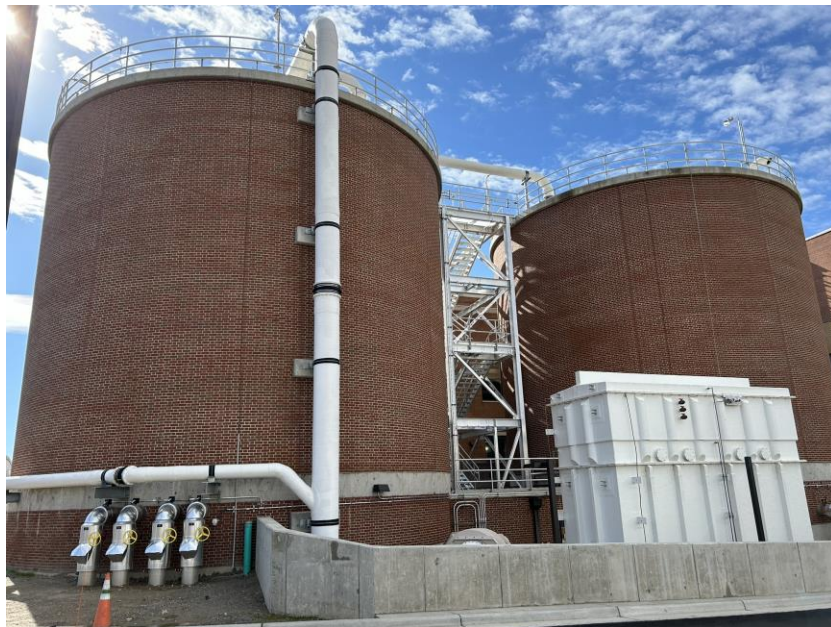
Figure 2-29: New R1 and R2 Sludge Storage Tanks
