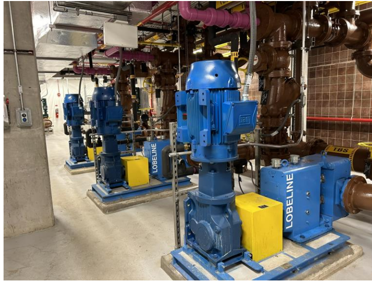
Figure 2-30: New R1 Centrifuge Feed Pumps
