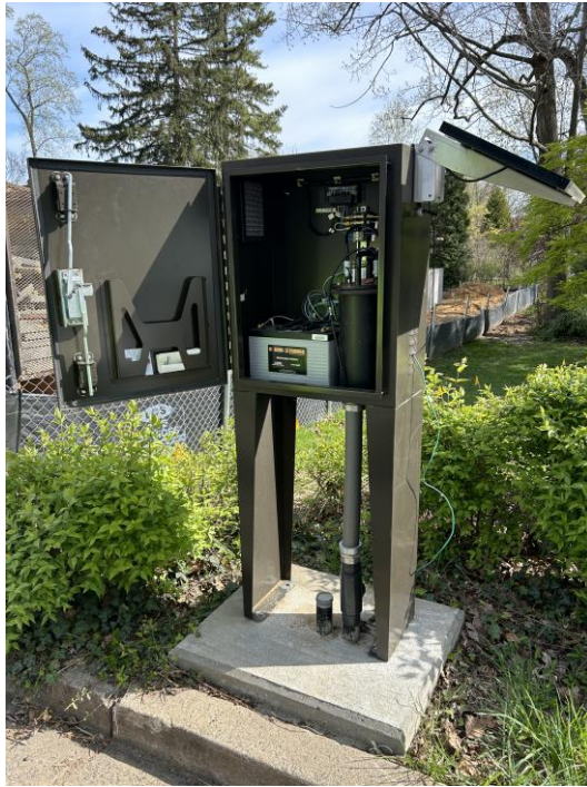
Figure 2-15: Tod Street Flow Metering Station
