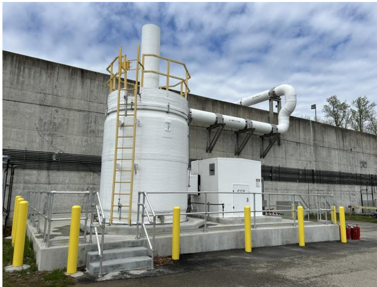
Figure 2-27: B3 Equalization Tank Odor Control Measures
