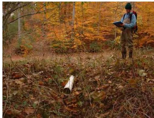
Photo 3.16 A storm drain pipe outfall is causing moderate erosion
