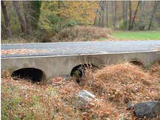
Photo 3.19 A culvert at (PHPH005.C001) Dunquin Court has a minor impact on the stream
