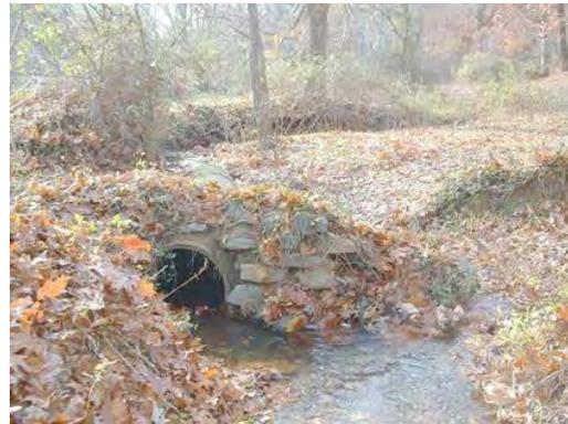
*Photo 3.11 A culvert (PHCC004.C002) at Wandering Lane has a moderate impact on the stream*
