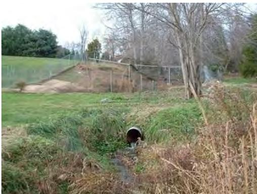
*Photo 3.12 A storm drain outfall pipe near Wandering Lane has a moderate impact on the stream*
