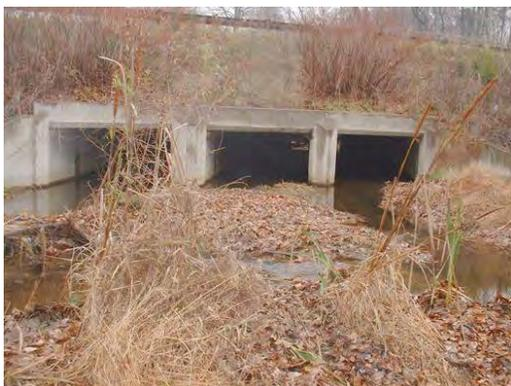
*Photo 3.1 A triple box culvert (PHPH044.C001) has at Braddock Road has a severe impact on the stream*
