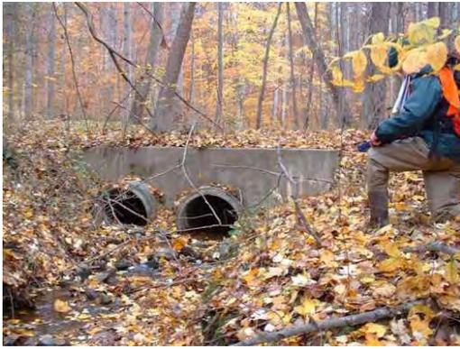
Photo 3.13 A double barrel culvert (PHPH025.C002) near Havenner Court has a minor impact on the stream
