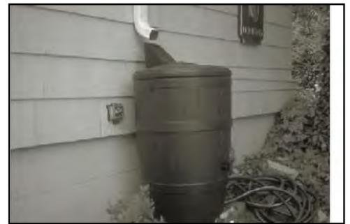
Figure 4.8: Rain barrel
