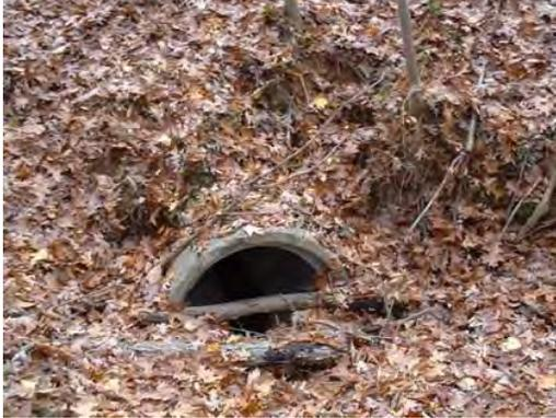
*Photo 3.8 A culvert (PHCC004.C008) at Knollbrook Drive has a moderate impact on the stream*
