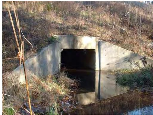
*Photo 3.7 A box culvert (PHPH028.C003) near Fairfax County Parkway has a minor impact on the stream*
