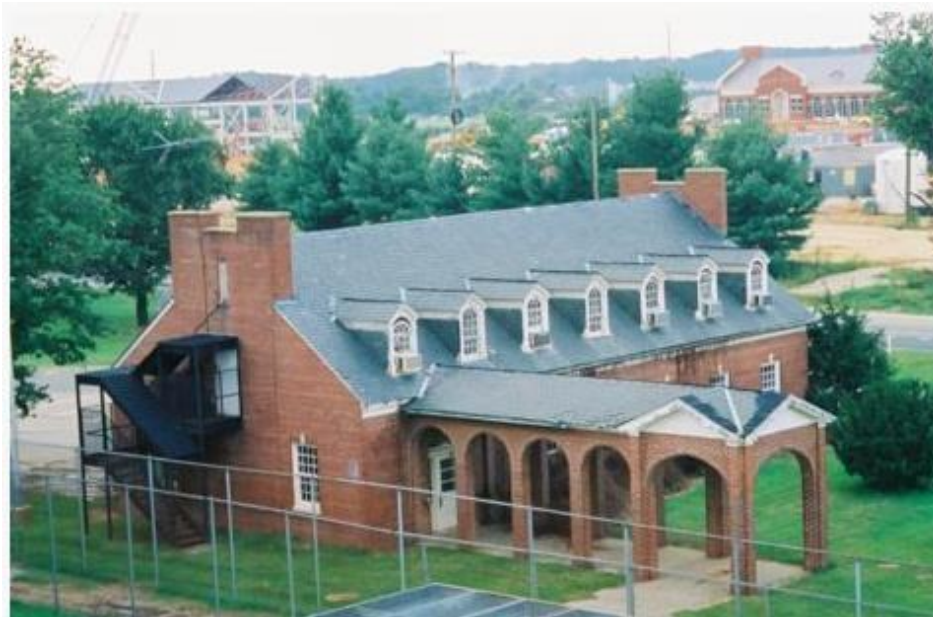
Workhouse Campus Building W15
