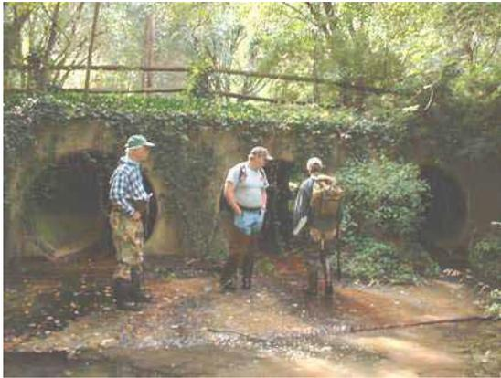
Photo 3.30 Triple 60" corrugated metal pipe culverts located under Davenport Street
