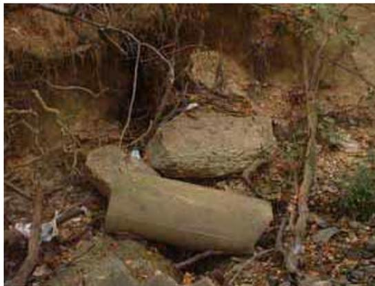
Photo 3.19 Severe erosion caused by discharge from an 18" pipe outfall west of the Mary Baldwin Drive crossing
