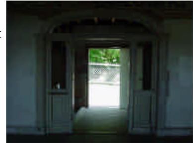
common in this area until after 1800. The stiles of the entrance are basically the pilaster types, although the reeding within the pilaster is rounded rather than flat. An opposing door at the north facade of the main block also was originally an exterior entrance but is now incorporated in the later addition. The keystone over the fanlight has a beaded center portion, which is similar to those found in the work of 19th-century architect Asher Benjamin.
