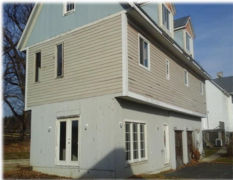
Figure 15: Turner Farm Garage with Apartment
