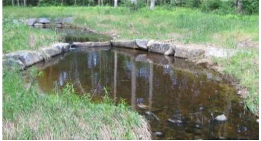
Reinforced Bed & Riffle Grade Control
