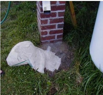
**Step 3.** Rain barrels need to be higher than ground level. A higher barrel = higher water pressure. Use bricks, cinder blocks, or pressure treated wood to create a platform.
