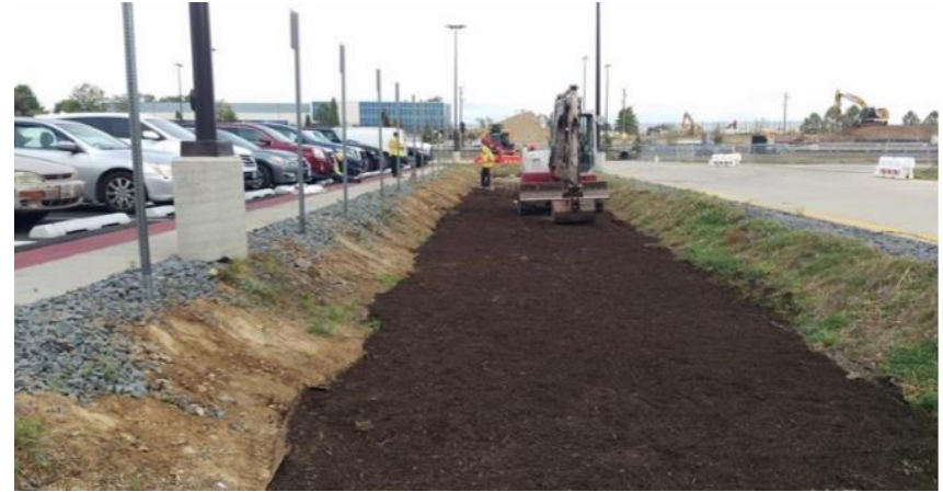
Grading in Bio Pond Water Quality Structure
