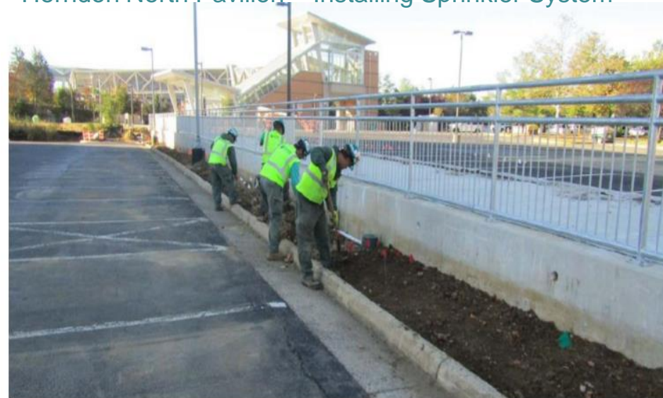
Herndon North Pavilion – Installing Sprinkler System
