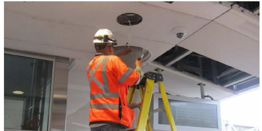
Installing Speakers in Ceiling Panels at Reston Station
