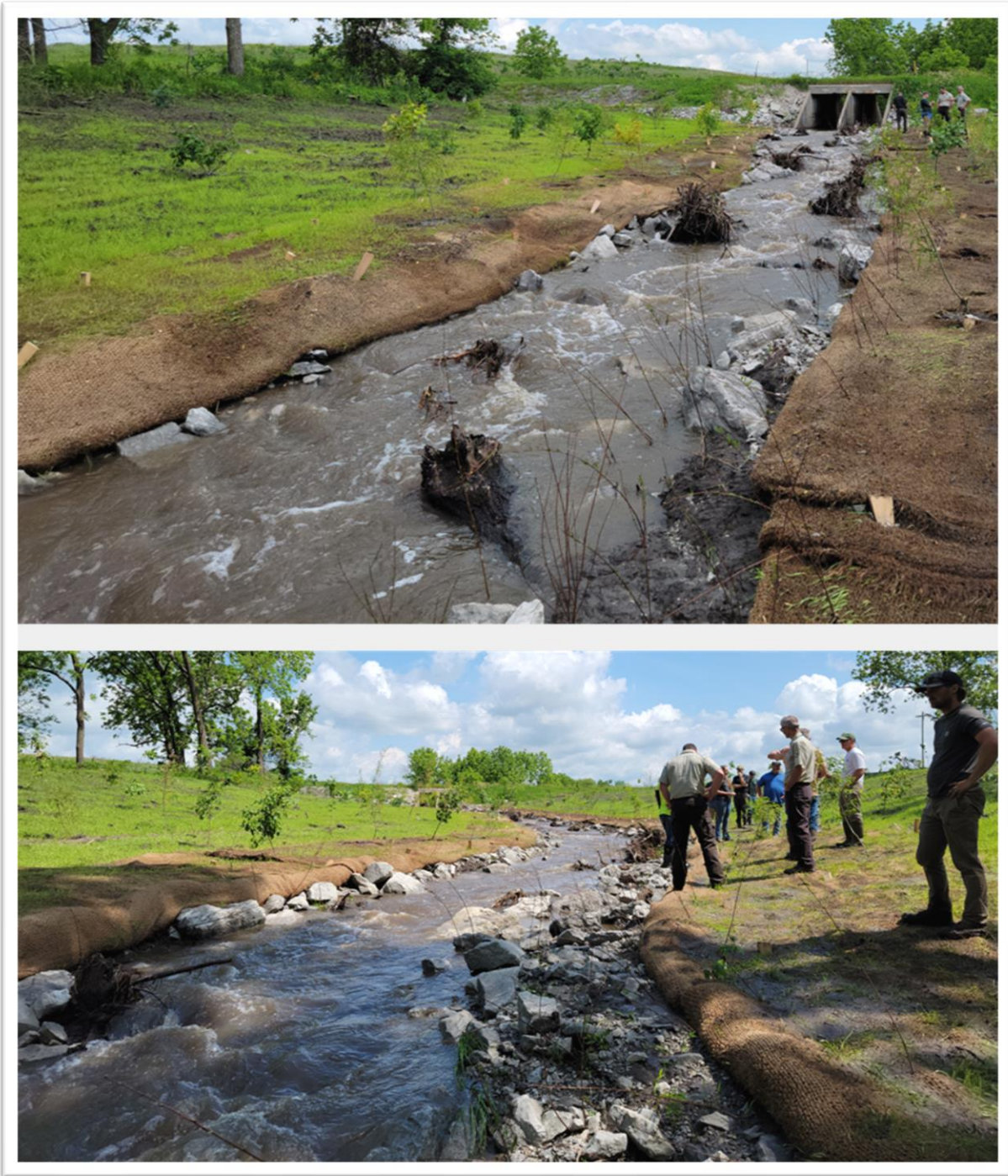
Figure 4-2 Little Creek rock ramp fish passage structure
