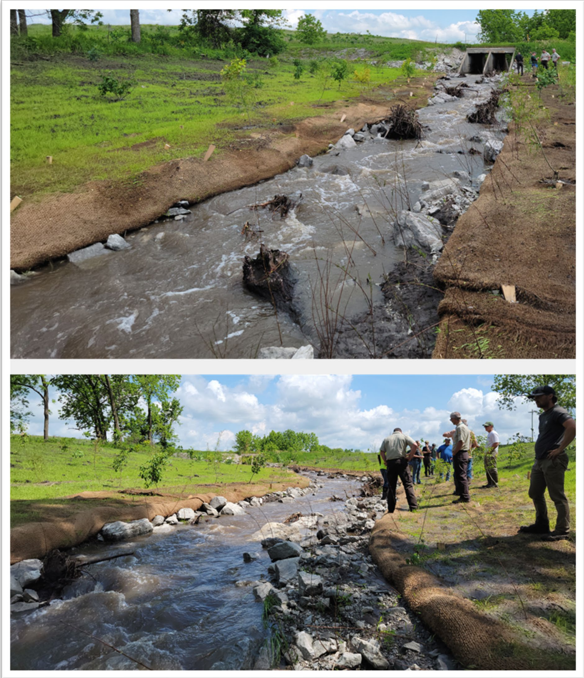
Figure 4-2. Little Creek rock ramp fish passage structure
