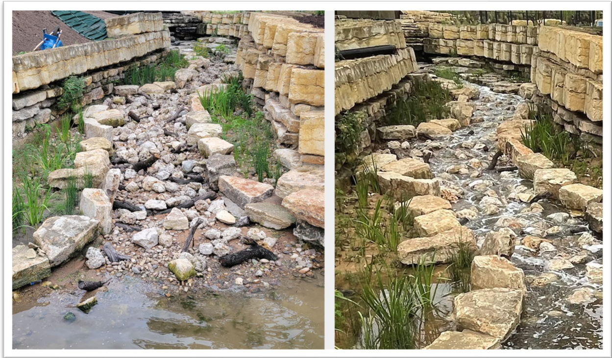
Figure 4-3. Waterloo Park Riffle Run rock ramp fish passage structure
