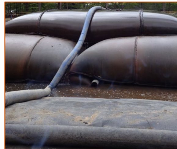
Step 3: Sediment Dewatering
