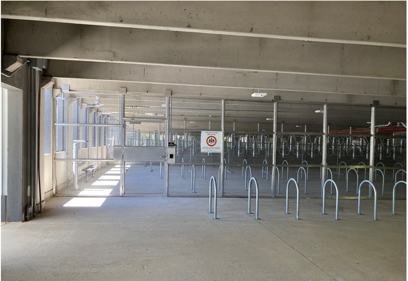
Bike room with controlled access
