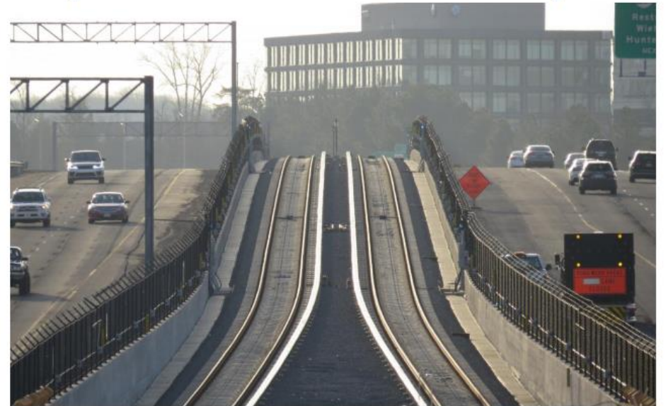
Guideway East of Innovation Station Ready for Testing
