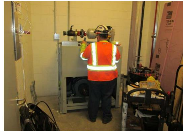
Installing Hydraulic Elevator Pump in MWB
