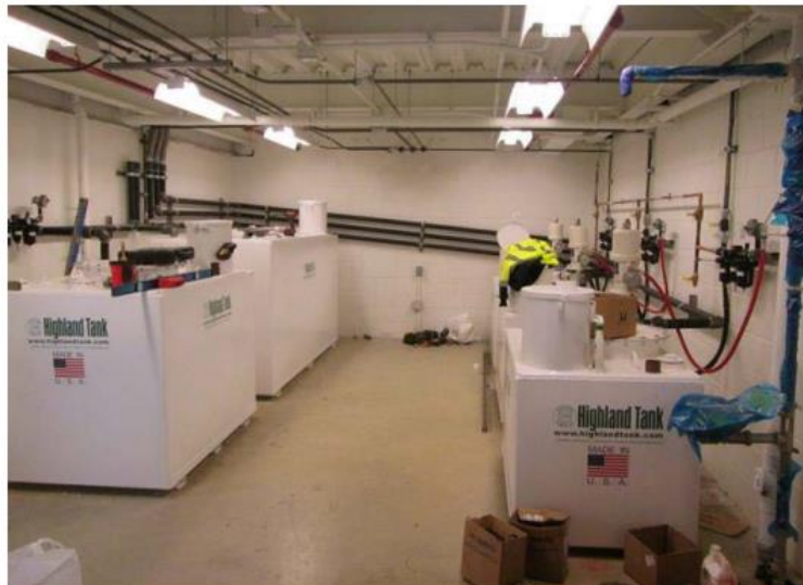
Lubrication Tank Room in MWB
