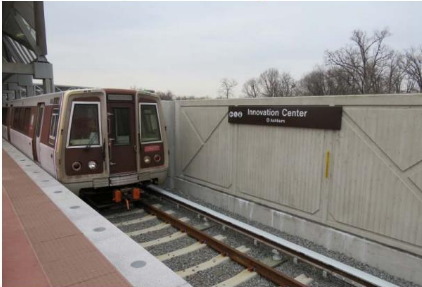
First Test Trains for Dynamic Testing on Phase Two Guideway
