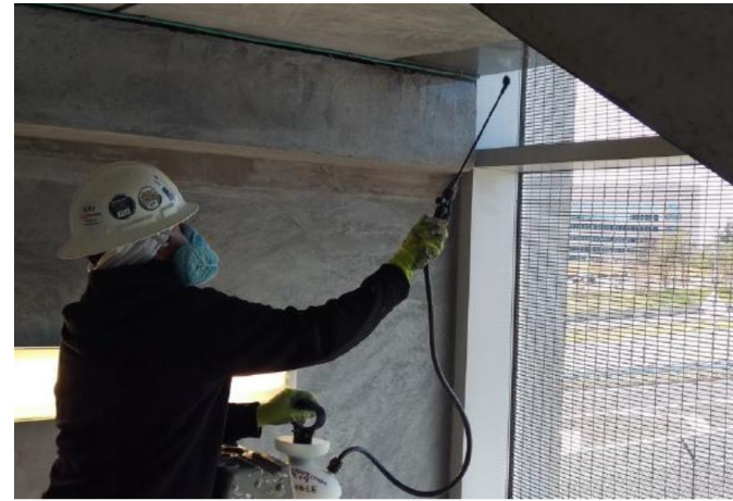
Applying Precast Sealant at Innovation Center Station Stair Tower
