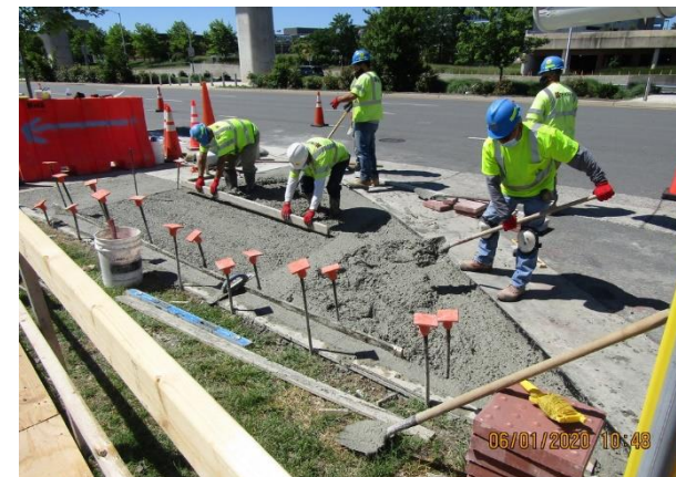
ADA ramp reconstruction along Route 7
