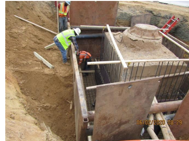
Communications vault work at Old Meadow Road
