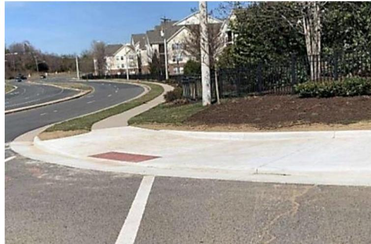
Suburban sidewalks are designed to provide a functional and safe space to walk separate from traffic. The 5 ft width is a minimum standard to accommodate wheelchairs. Trees, lighting and benches are not always provided.
