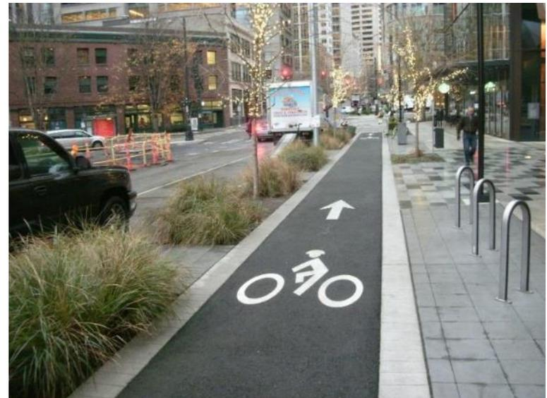
Separated bikeways, also known as protected bike lanes or cycletracks, provide a dedicated place for bicyclists to ride physically separated from pedestrians and from cars. Separated bikeways can be one-way on each side of the road, or two-way.
