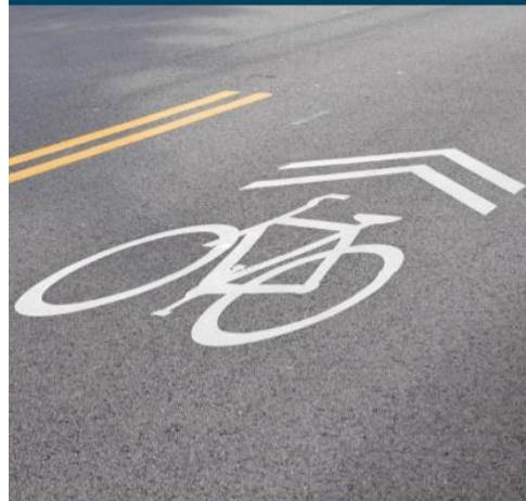
SHARED LANE MARKING (SHARROW)
