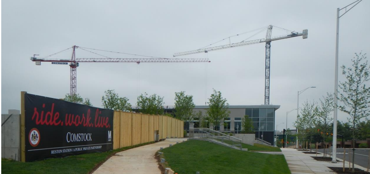
The Wiehle-Reston East Metrorail station, opening in 2014, will transform the Reston transportation network
