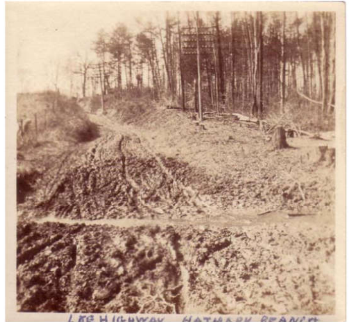
Lee Highway at Hatmark Branch, looking SW towards the Town of Fairfax, March 9, 1924. Note the creek flowing across Lee Highway. Blake Lane (not visible) is at the top of the hill. Photo courtesy of Lee Hubbard.
