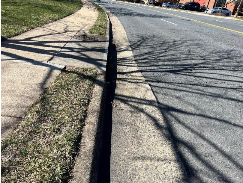
Figure 5: Pavement Inconsistency Southbound before Lightfoot Road
