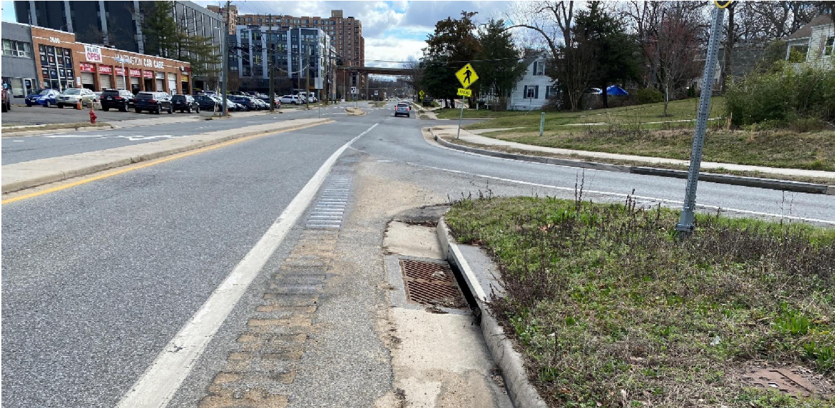
Figure 3: Curb inlet at access ramp between Telegraph Road and Kathryn Street
