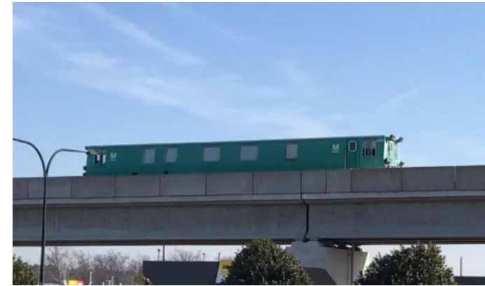
Track Geometry Vehicle on Aerial Guideway
