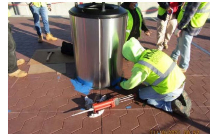
Trash Can Installation
