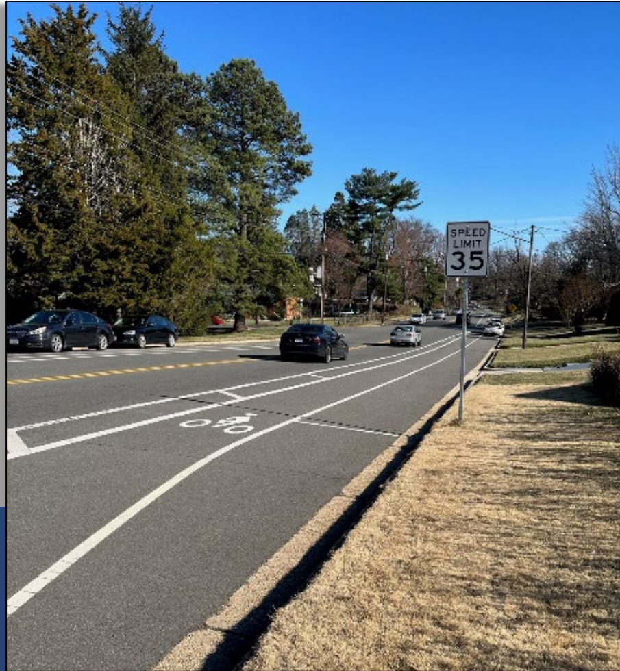
BLTS 2: Near Thornton St, southbound
