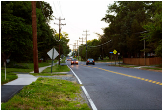
The uneven sidewalk along the west side of southbound Van Buren Street has frequent obstructions (utility pole and shrubs), which reduce the effective width for pedestrians. Similar obstructions or gaps in the existing sidewalk network are opportunities to improve pedestrian connectivity.
