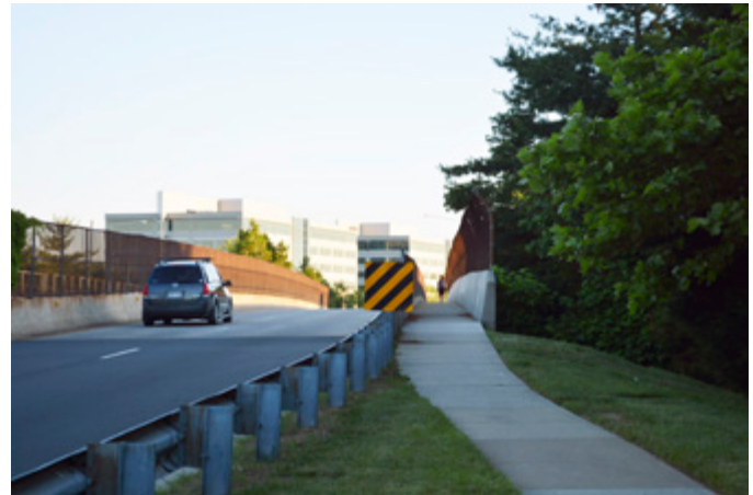
Pedestrian accommodations on west side of Monroe Street bridge. The Monroe Street crossing of the Dulles Toll Road is the only crossing in the study area without interchange ramps, making this location an attractive crossing for pedestrians and bicycles due to lack of conflicts with turning traffic.
