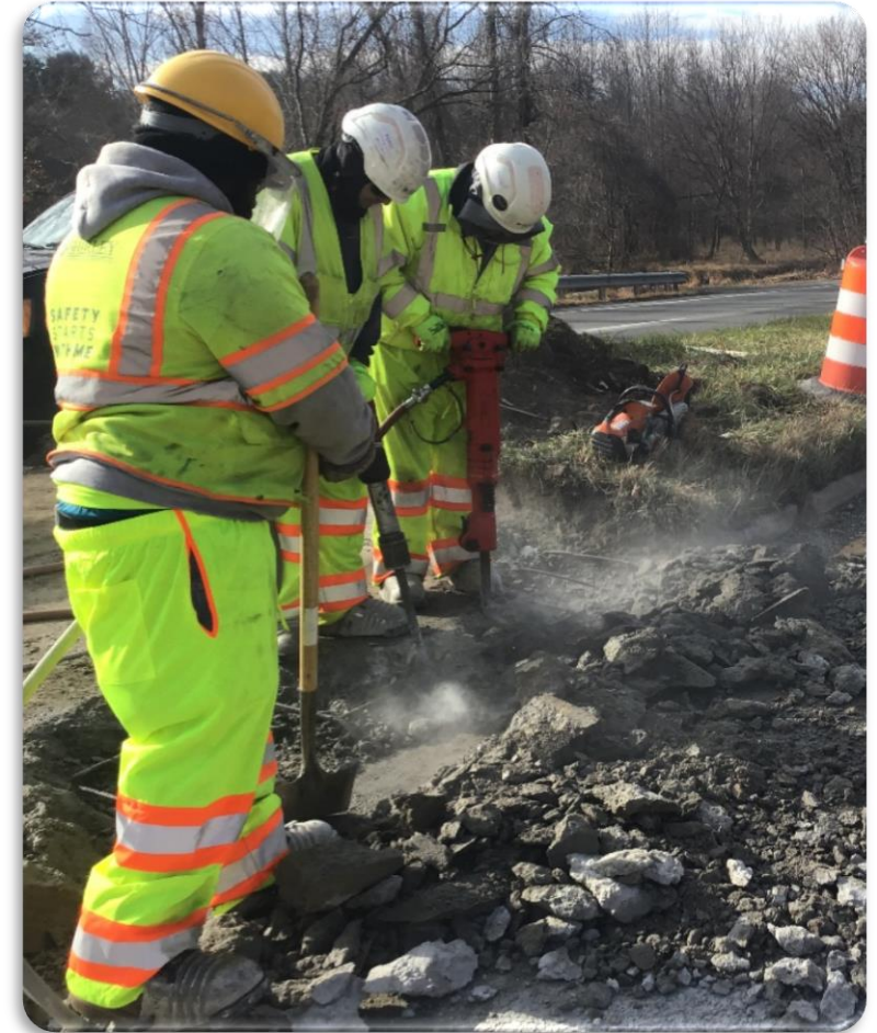
Crew removing Raised Median
