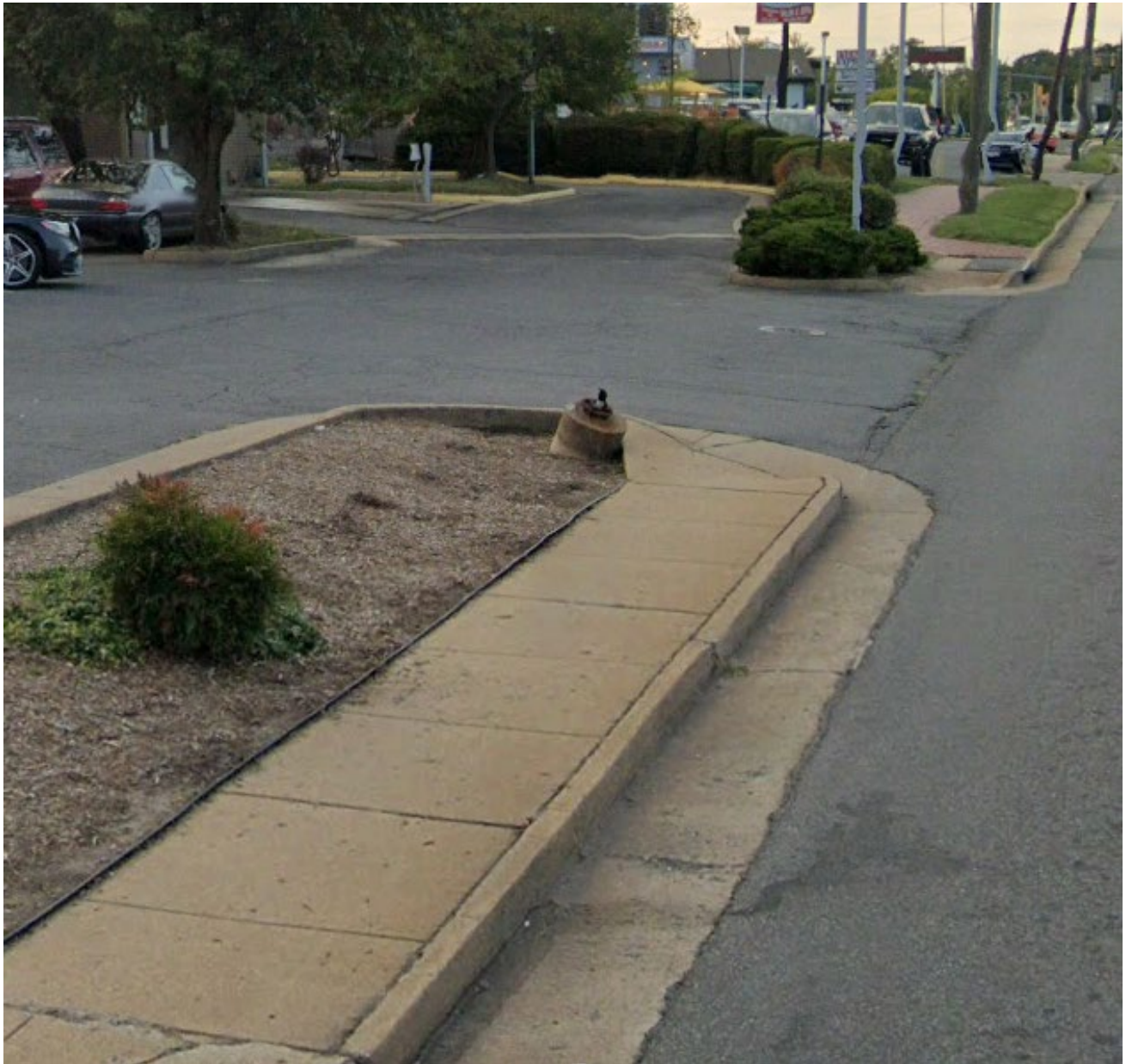
Image 4-2: Sidewalk on Route 7 Approaching Interchange
