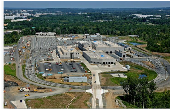
Dulles Rail Yard
