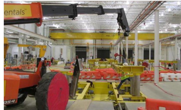
Hoist Installation in SIB
