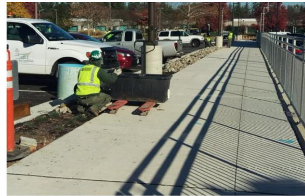
Placing River Rock at Herndon North Pavilion
