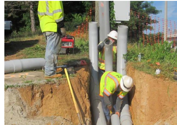
Conduit installation and tie-in
