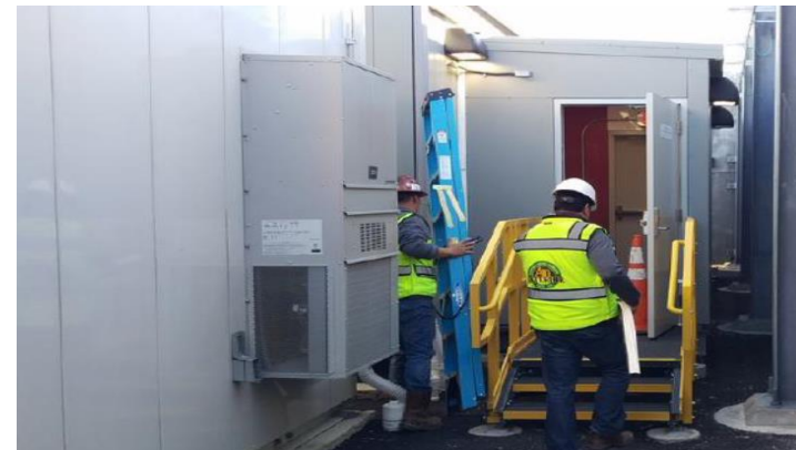
Tie Breaker Station (TBS) #16 Exterior Enclosure
