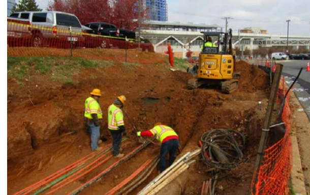
Cable installation
