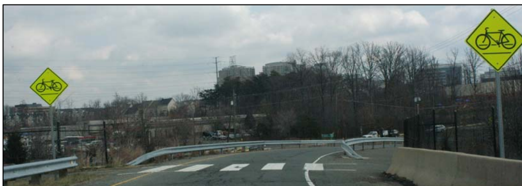
Figure 3-16: Fairfax County Parkway Trail crossing at Sunset Hills Rd.
