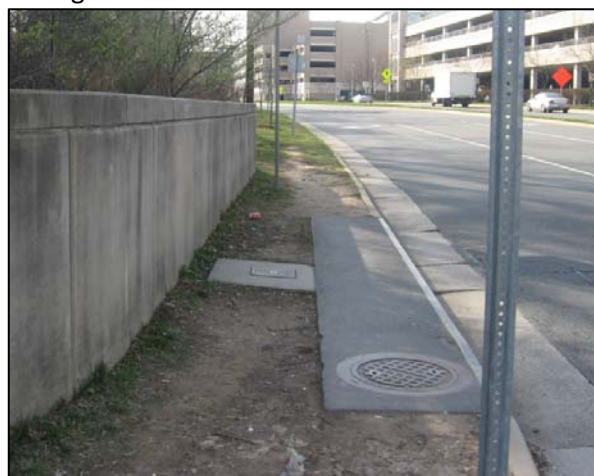
Figure 3-12: Missing sidewalk on Bluemont Way near Reston Parkway.
