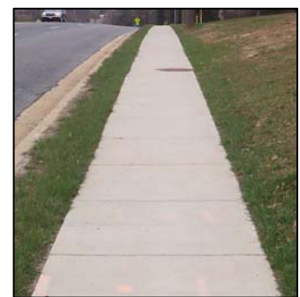
Figure 3-36: Sidewalk east of Plaza America
