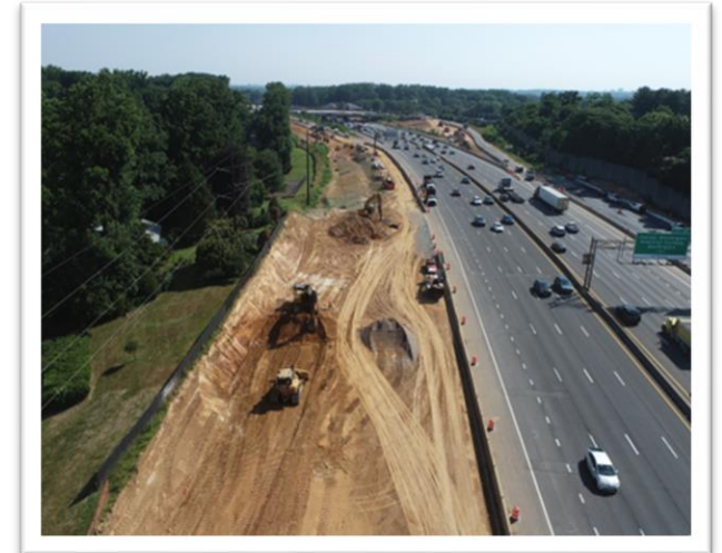
Top: Crews perform earthwork, enabling new outside lanes to be built (June 2024)
