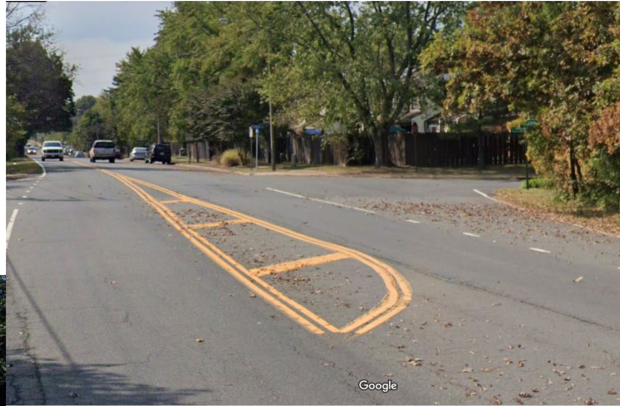
Crestview Drive Facing South Approaching Ferris Avenue on the Right
